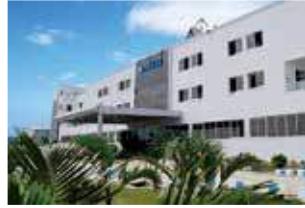
Rudrapur Plant (Green Building)
