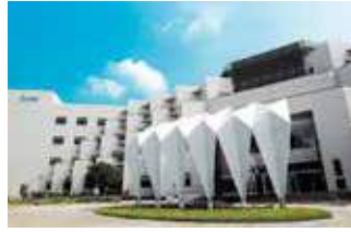
Tainan Plant (Diamond-rated Green Building)
